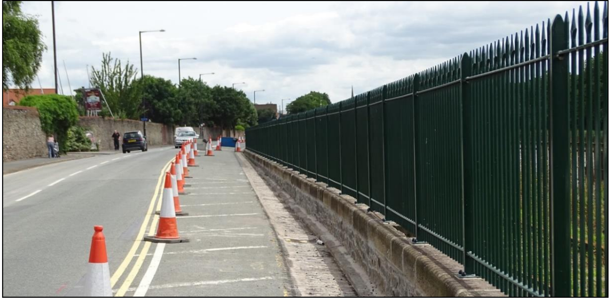
Figure 17 - The MetroBus flood wall on Cumberland Road
