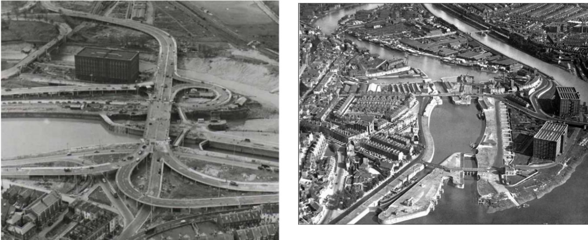
Figure 16 - Construction of Junction Lock, 1964 (left) and Brunel Harbour, 1929 (right)
