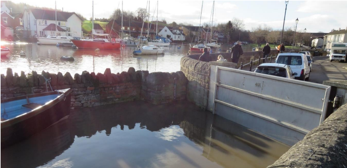
Figure 20 – Existing flood defences in operation at Pill
